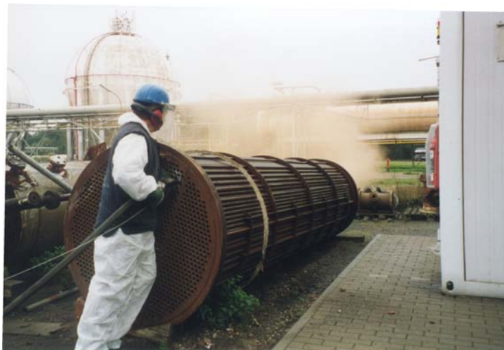
Fig. 4: Cleaning a heat exchanger using the CryoClean® process
